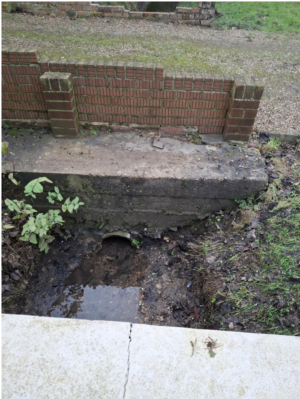
(Photograph 4 - Drainage ditch heavily accumulated with silt on Folkingham Road) (Taken by GeoSmart Consultant, 12 February 2025).
