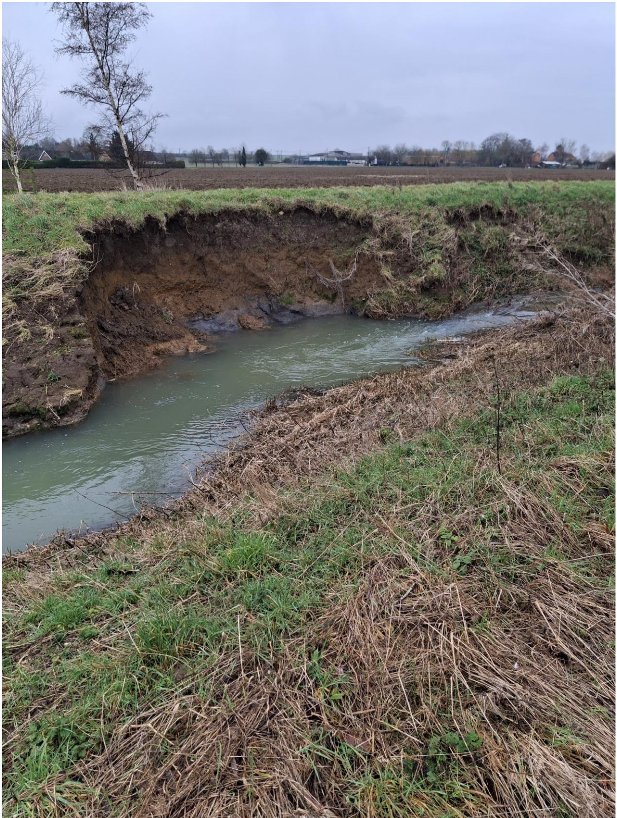
Photograph 7 – Subsidence of embankment) (Taken by GeoSmart Consultant, 12 February 2025).
