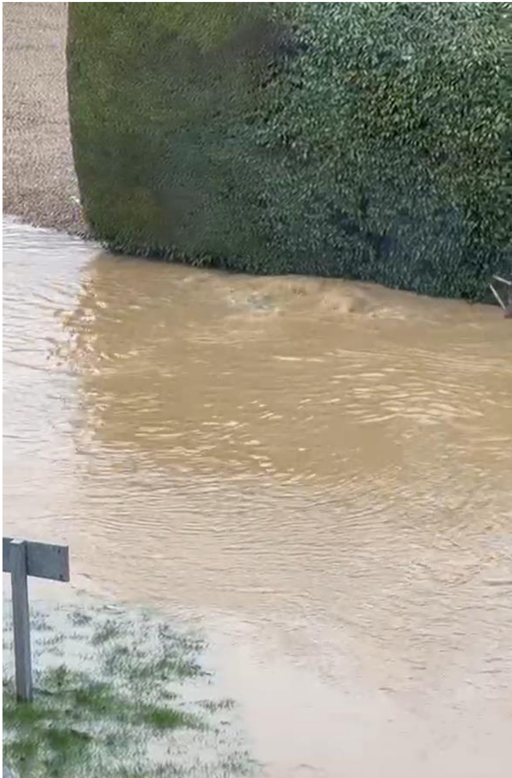
(Figure 22 - Surcharging manhole cover within Vine Court) (Taken by Billingborough resident, 06 January, 2025).
