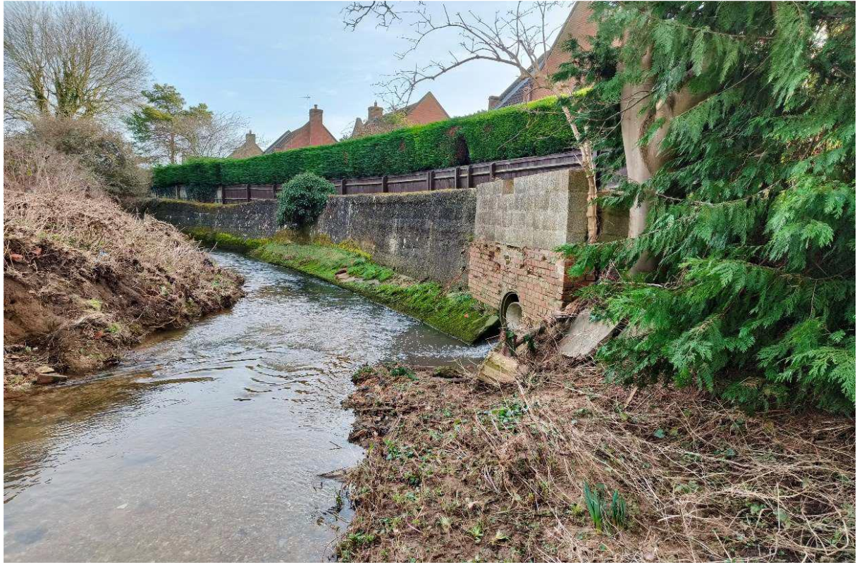
(Figure 21 - Surface water drainage discharge outlet into Ousemere Lode) (Taken by Billingborough resident, date unknown).
